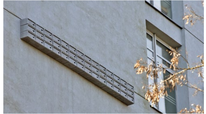
Swift nesting boxes mounted on the building of the Institute of Architecture and Urban Planning. Source: TUL archive
